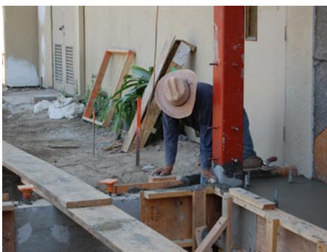
*Jose Moreno trowels the concrete around the elevator structure and on top of the footings giving it a smooth surface.*
