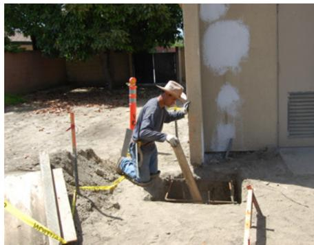
*Jose Moreno, concrete finisher stamps down the concrete in the canopy footing to fill in the voids.*
