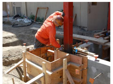
*Vibrating the concrete in the elevator structure footing to help it settle and remove air voids.*
