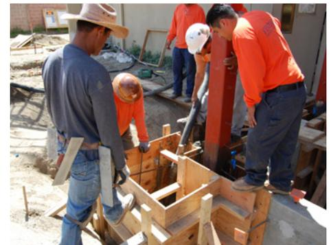
*Pumping concrete into the elevator structure footing.*
